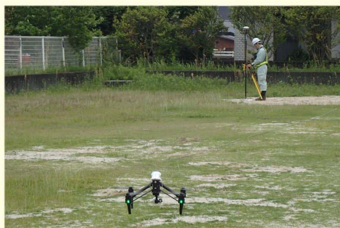
i-Construction ( ICT土工 ) 研修
